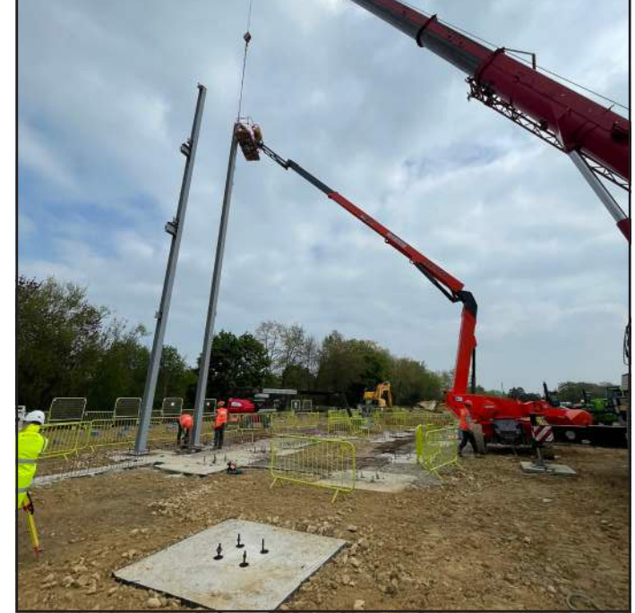
Steel deliveries will continue for a few weeks
