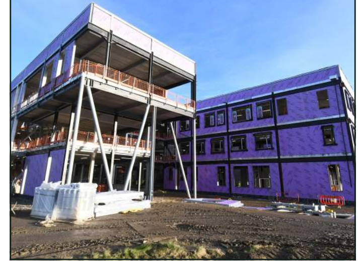
External cladding going in
