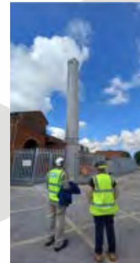
Replacement of Coal fired boilers at Goole District Hospital with gas fired steam raising boilers
